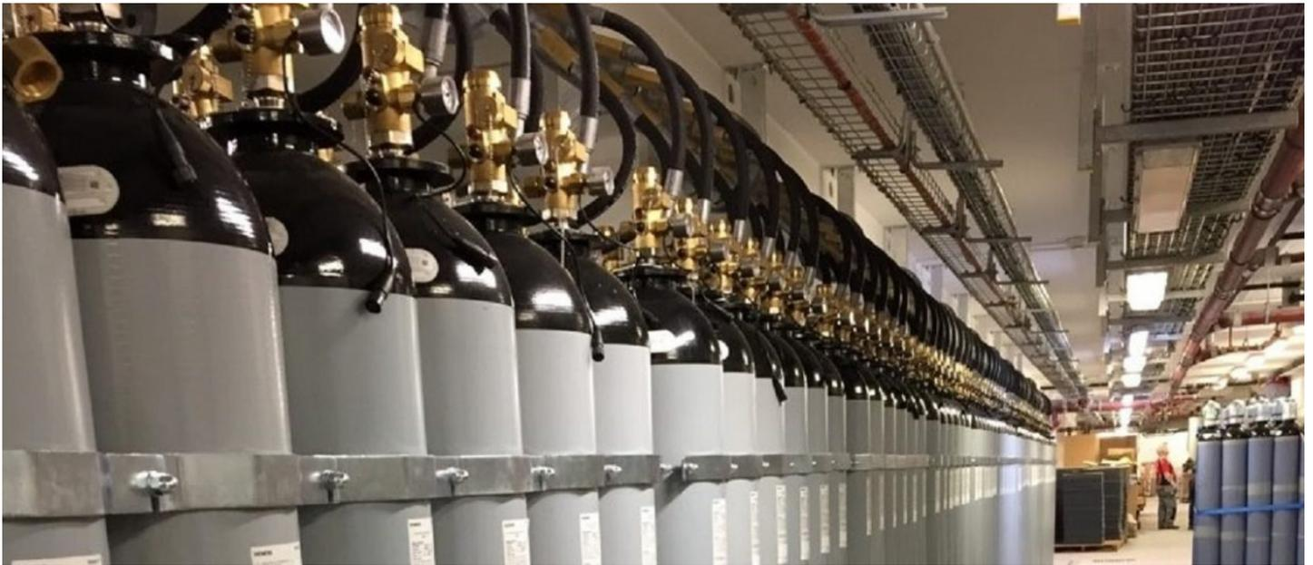
A gas system protects enclosed areas and works by totally flooding the area, with the exception of with CO<sub>2</sub> which can protect an object by local application.
